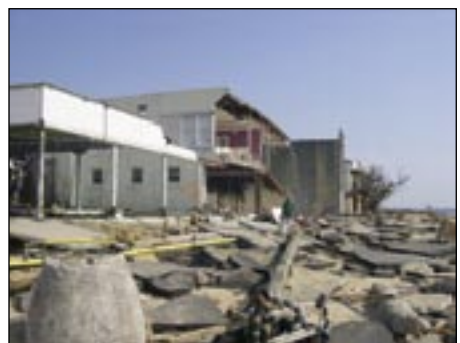
BEACH BOULEVARD IN BAY SAINT LOUIS SHOWING SOME OF THE REMAINING BUILDINGS AND WHAT USED TO BE THE ROAD BED.
