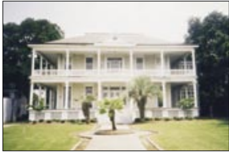
THE HISTORIC ROBINSON MALONEY DANTZLER HOUSE BEFORE KATRINA. ONLY THE FOUNDATION REMAINS ON BEACH BOULEVARD IN BILOXI.
